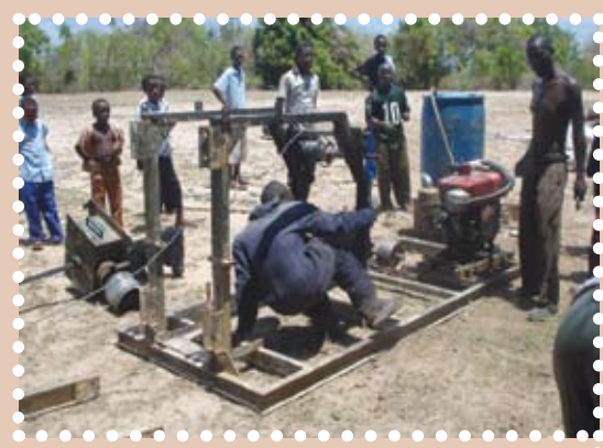
Set up of drilling equipment
