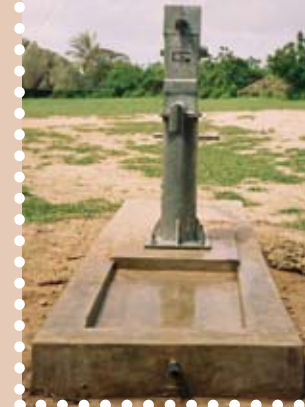
Hand pump installed
